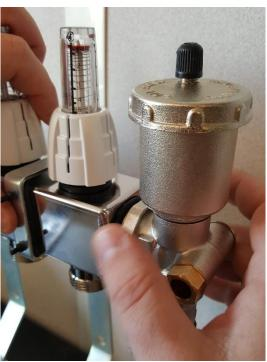
Engage the nut onto the thread and then use a key to compress the oring seal while maintaining the purge module in a vertical position with a second key.
